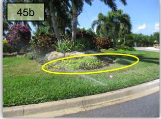
46. I also flagged several MP Rotator heads on the WLBIvd. median between Field Brook and the roundabout that were either not popping up, popping up but not spraying anything out or popping up and not turning. Some other were not turning a full 180° but stopping short of the curb causing turf to stress. In all areas where MP Rotators were not operating properly, turf and plants were dying.
